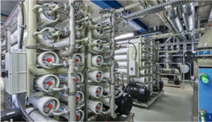
1 Membrantrennanlage – GAW water technologies.
